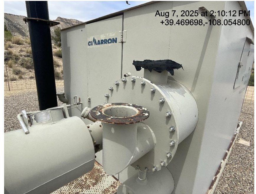
Photo # 9461 Burner exhaust open ended/wildlife hazard /available for entry by wildlife
