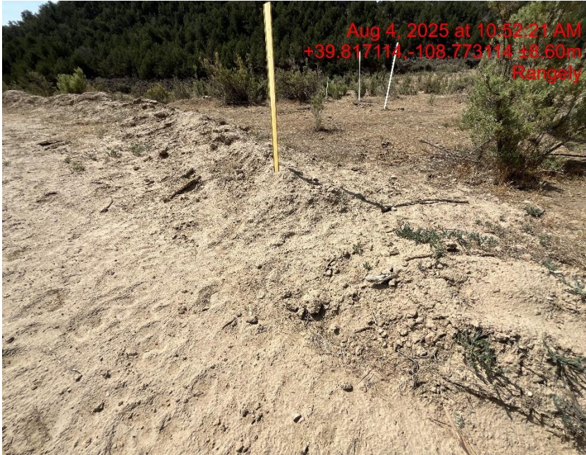
Photo # 1225 Berms on location need maintenance
