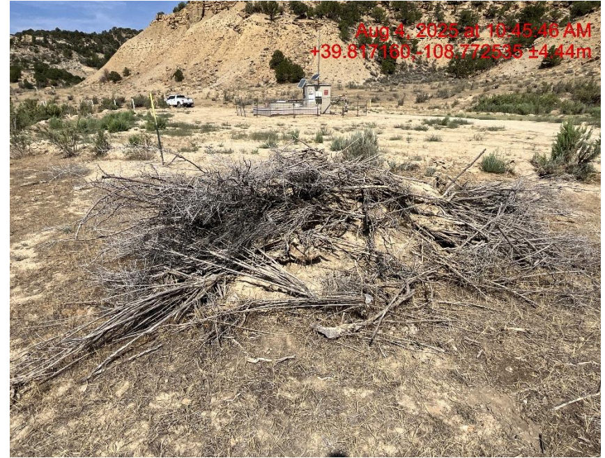
Photo # 1217 Stockpiled soils with no BMP's from other side
