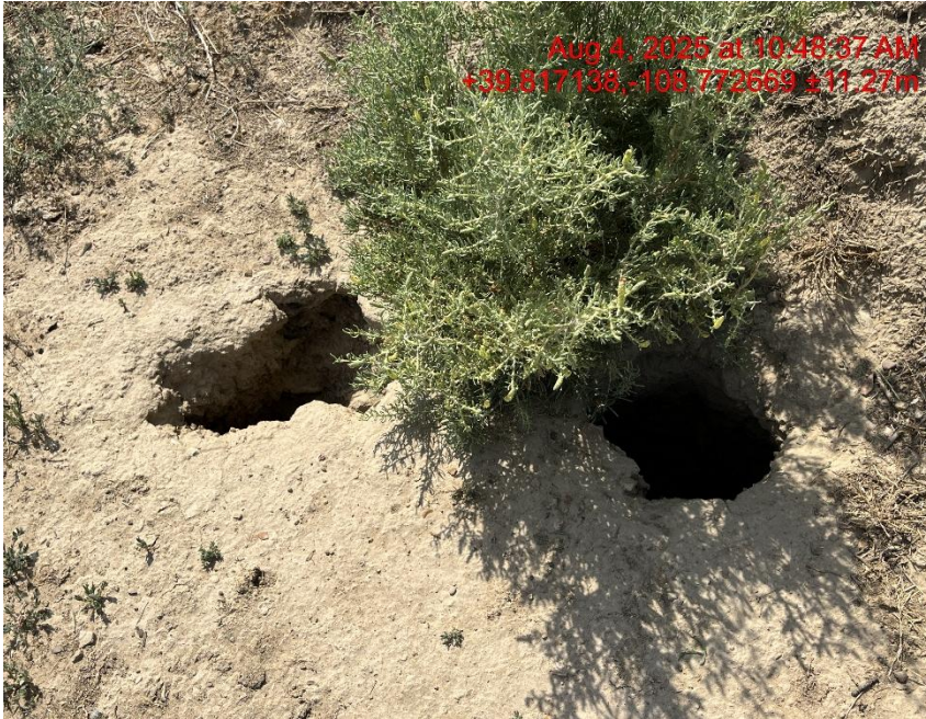
Photo # 1219 Tunnel erosion on south side of location is a wildlife hazard/personnel safety hazard
