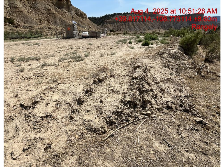
Photo # 1224 Berms on location need maintenance
