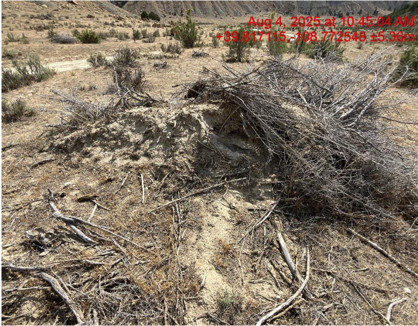
Photo # 1216 Stockpiled soils with no BMP's
