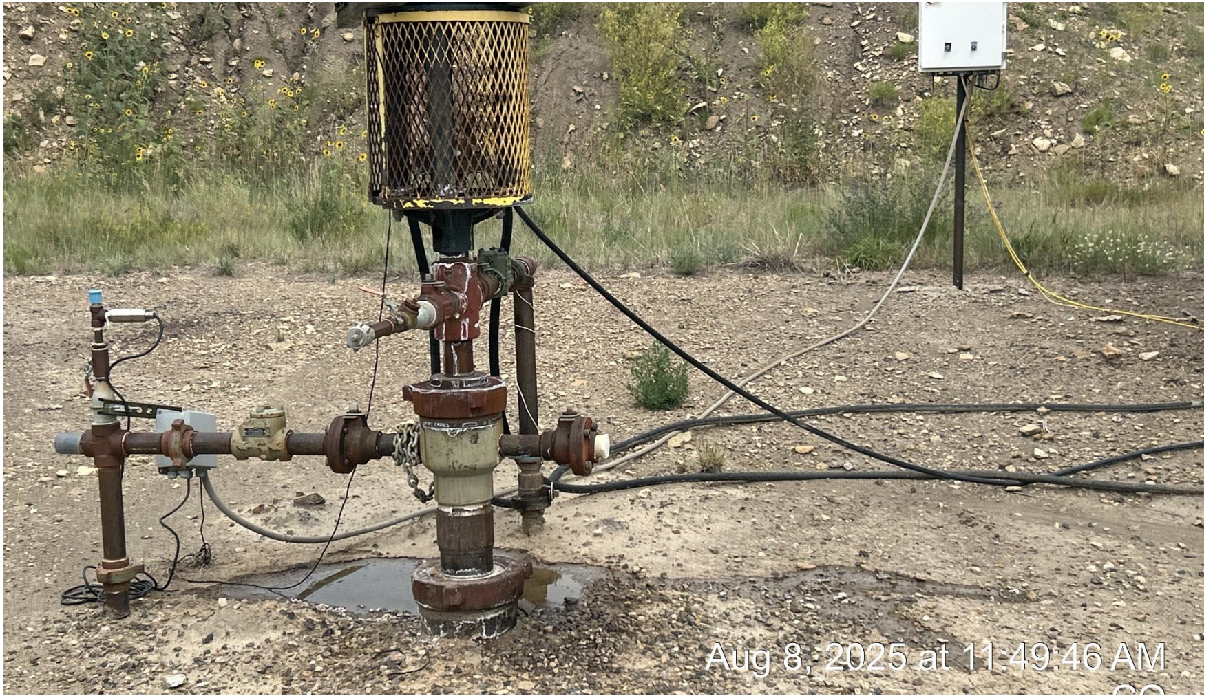
PHOTO 2: LOCATION – PACKING LEAK
