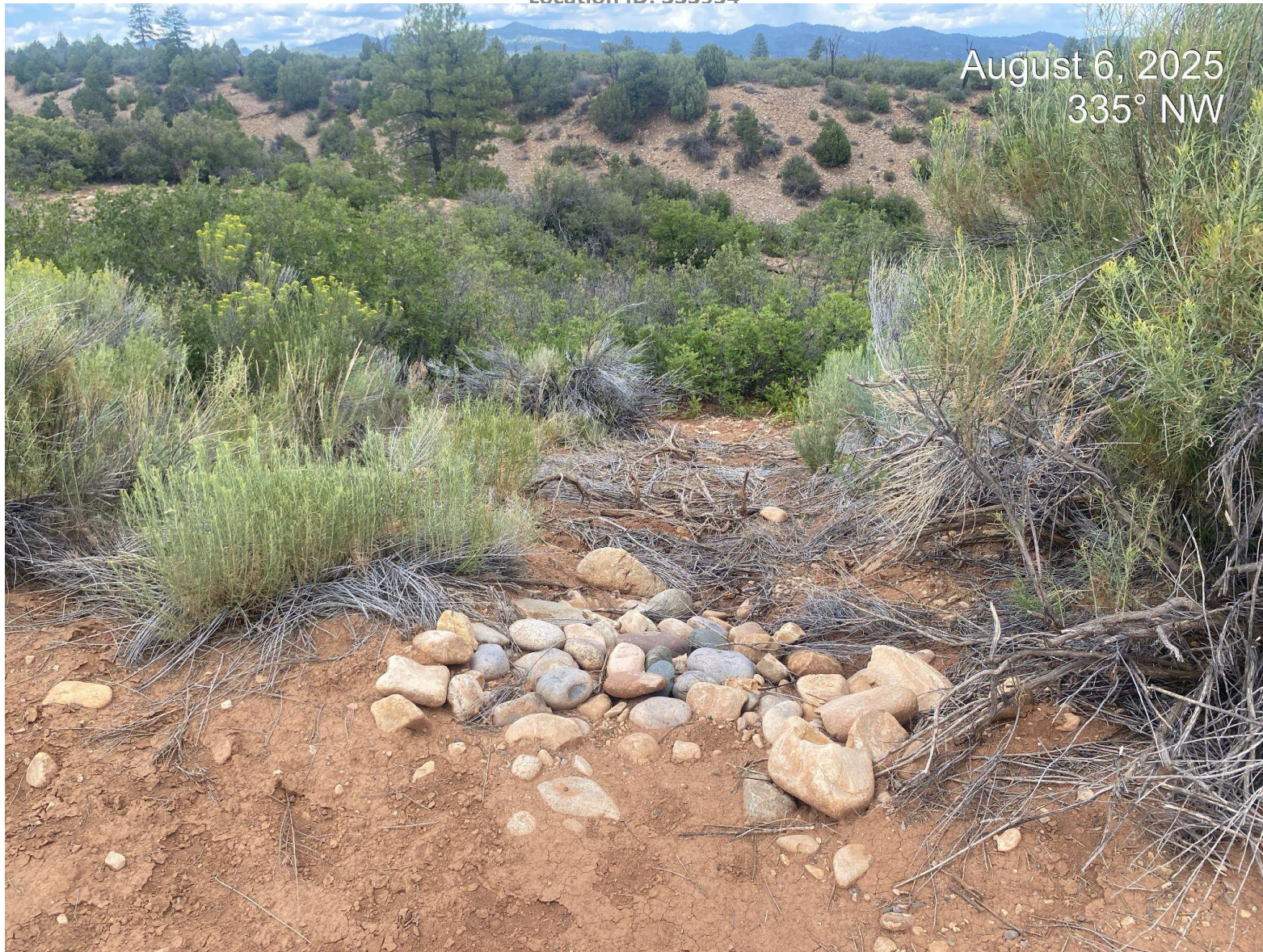
Photo 2. Stormwater BMPs have been installed in previous gully erosion area, erosion appears to be controlled at this time.
