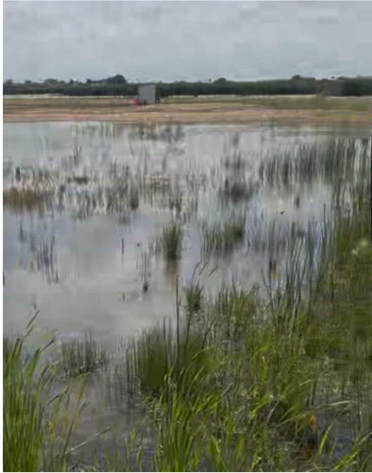
Photo Taken Facing Southeast from Access Road Toward Meter House
