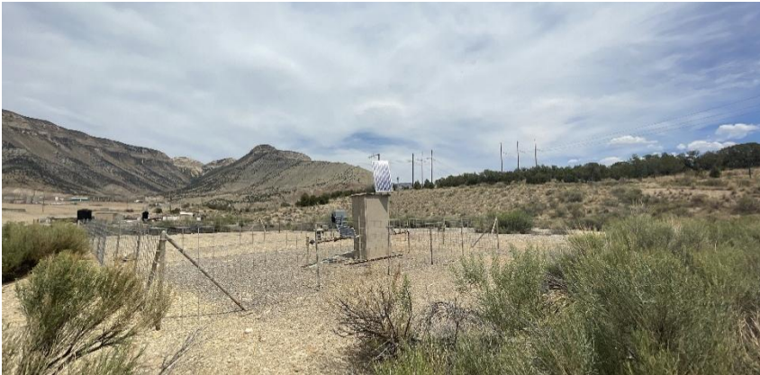
South West corner of location.
