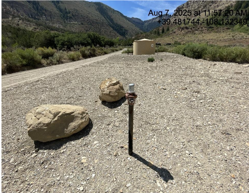
Photo # 9133 Unused flowline lacks lockout tagout (OOSLAT)
