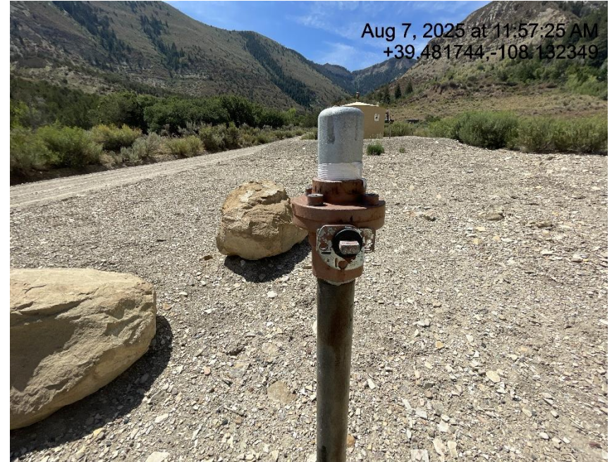
Photo # 9134 Unused flowline lacks lockout tagout (OOSLAT)
