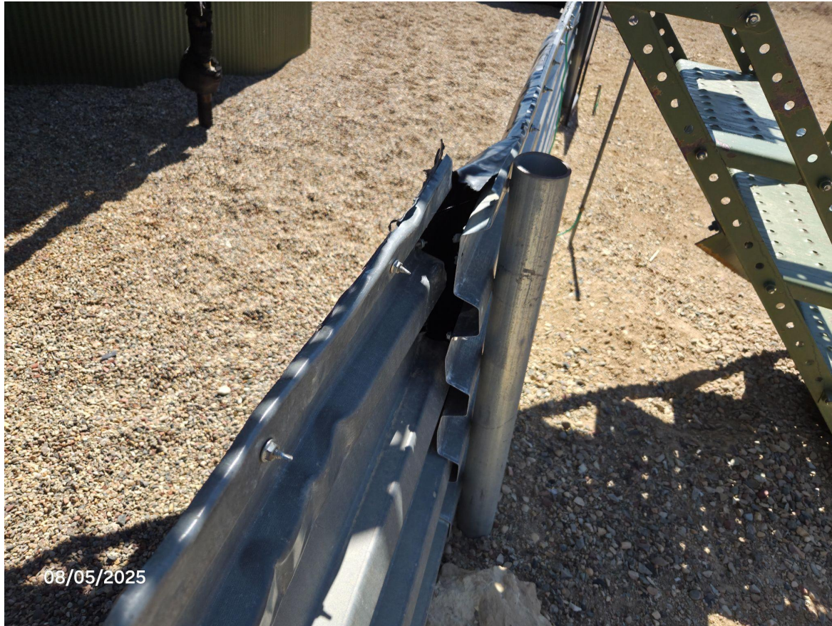
Photo 16: Photos 16-17 taken from the tank battery facility. Photo shows the metal berm has become separated.
