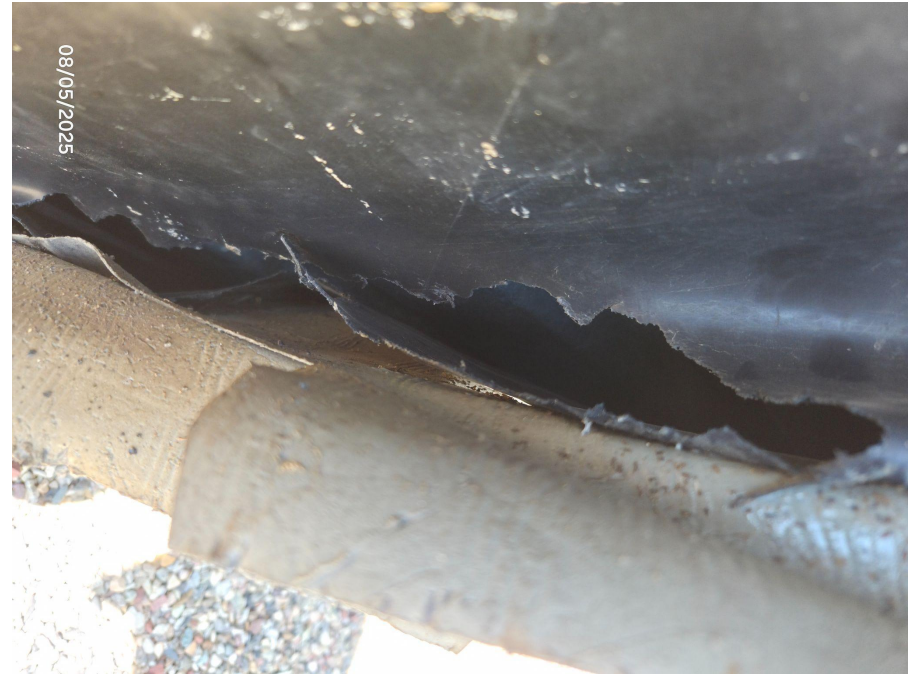
Photo 17: Photo shows tear observed within liner at the tank battery facility.
