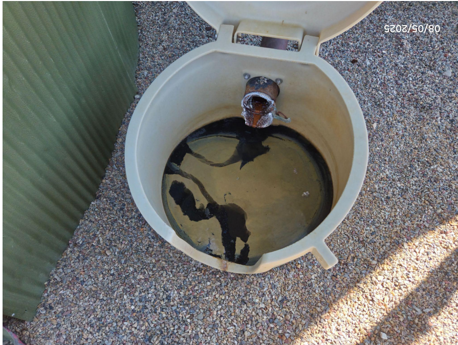
Photo 15: Photos taken from the battery facility. Photos show lines at tanks missing cap/plug. Photo left also shows fluids spilled within containment.
