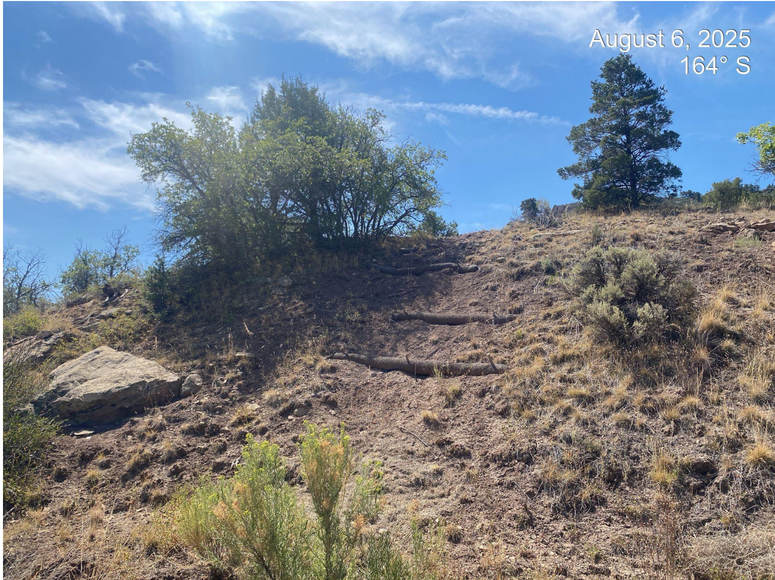
Photo 3. New stormwater BMPs installed on southern cut slope, appear to be functioning at this time.
