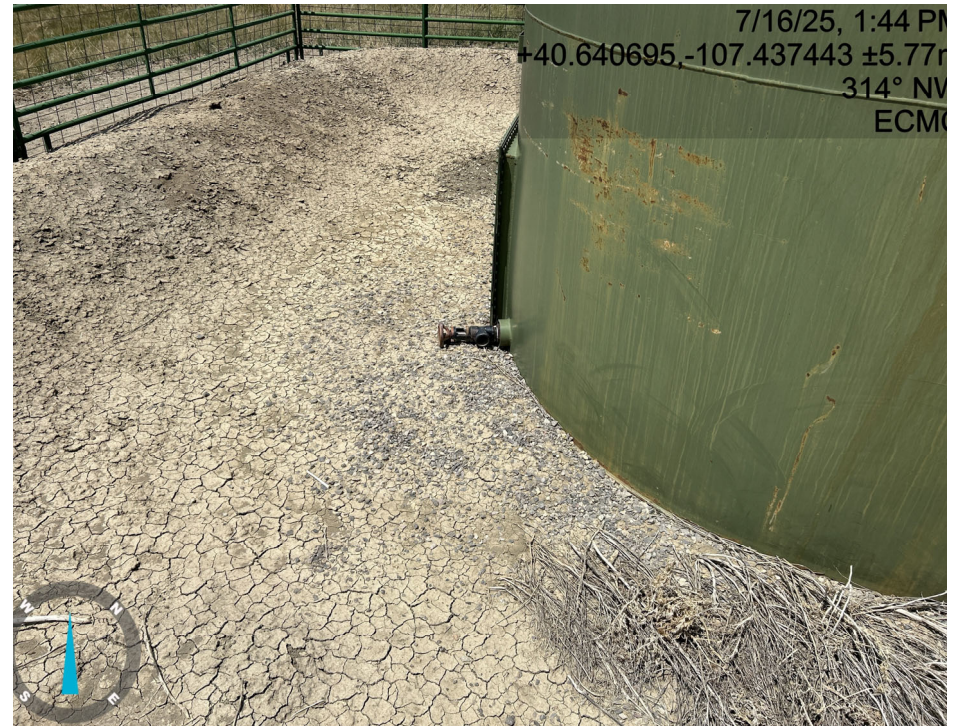
Load lines not plugged/capped
