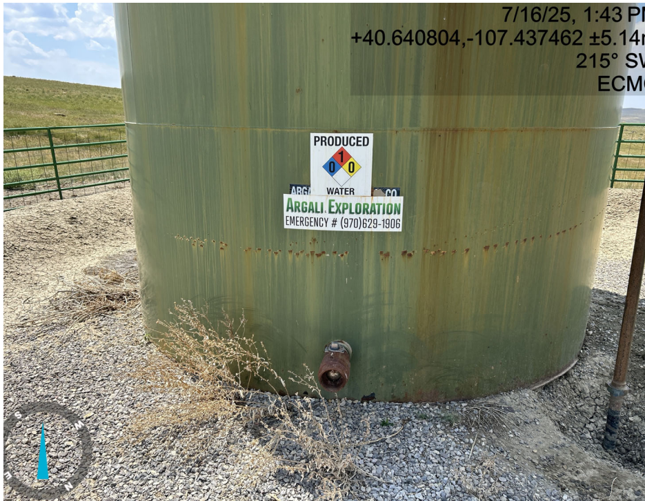
Load lines not plugged/capped also labeling lacks information
