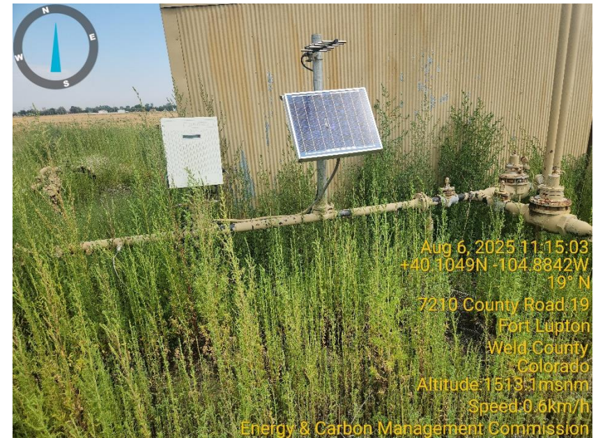
Photo 8 Gas Meter Run not currently calibrated & over grown with new vegetation on top of the dead vegetation.
