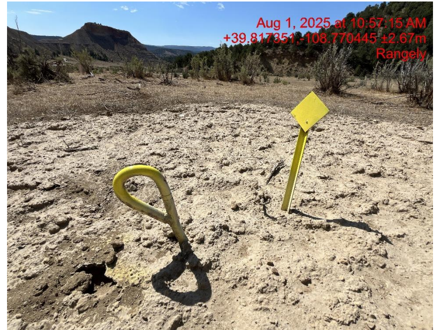
Photo # 1176 Improperly marked deadman
