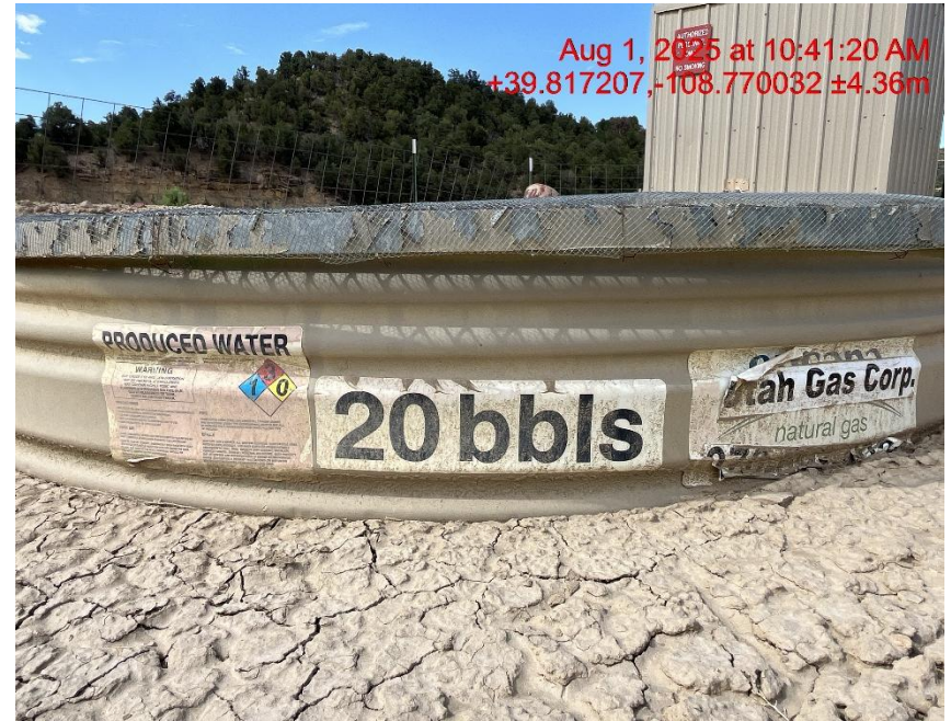
Photo # 1160 Tank lacks required labeling
