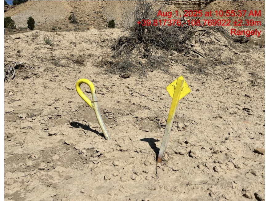
Photo # 1174 Improperly marked deadman
