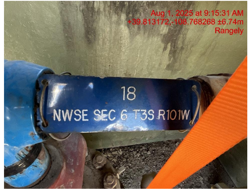
Photo # 1092 Wellhead sign lacks required information
