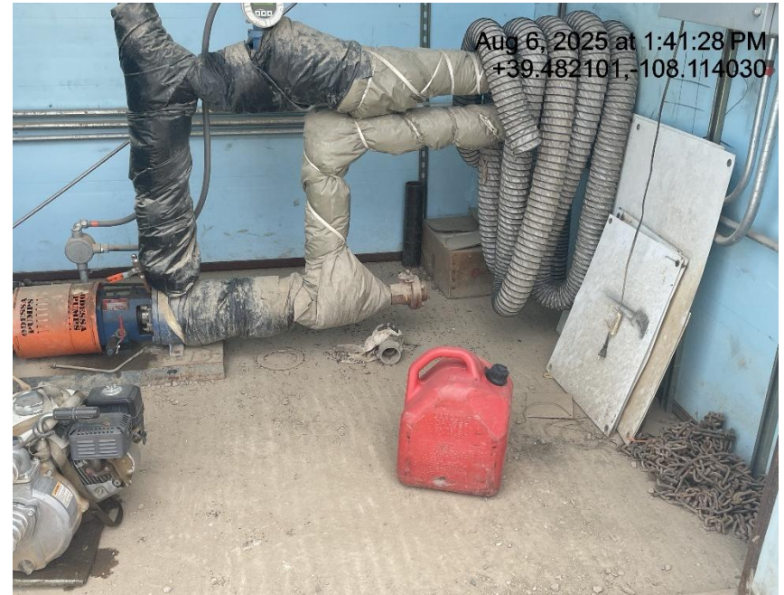
Photo # 8411 Improper storage of flammable liquids in shed/shed not in compliance with CECMC Rule 610
