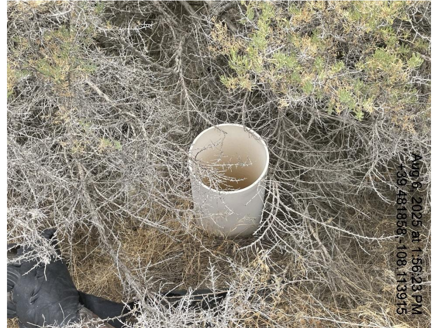
Photo # 8425 Open ended piping/wildlife hazard/available for entry by wildlife
