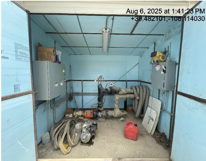
Photo # 8410 Improper storage of flammable liquids in shed/shed not in compliance with CECMC Rule 610
