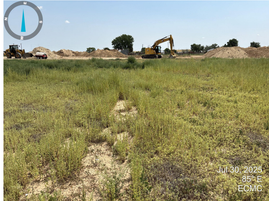
Photo 4. Looking east from the wellbore. See photo 2 comments.
