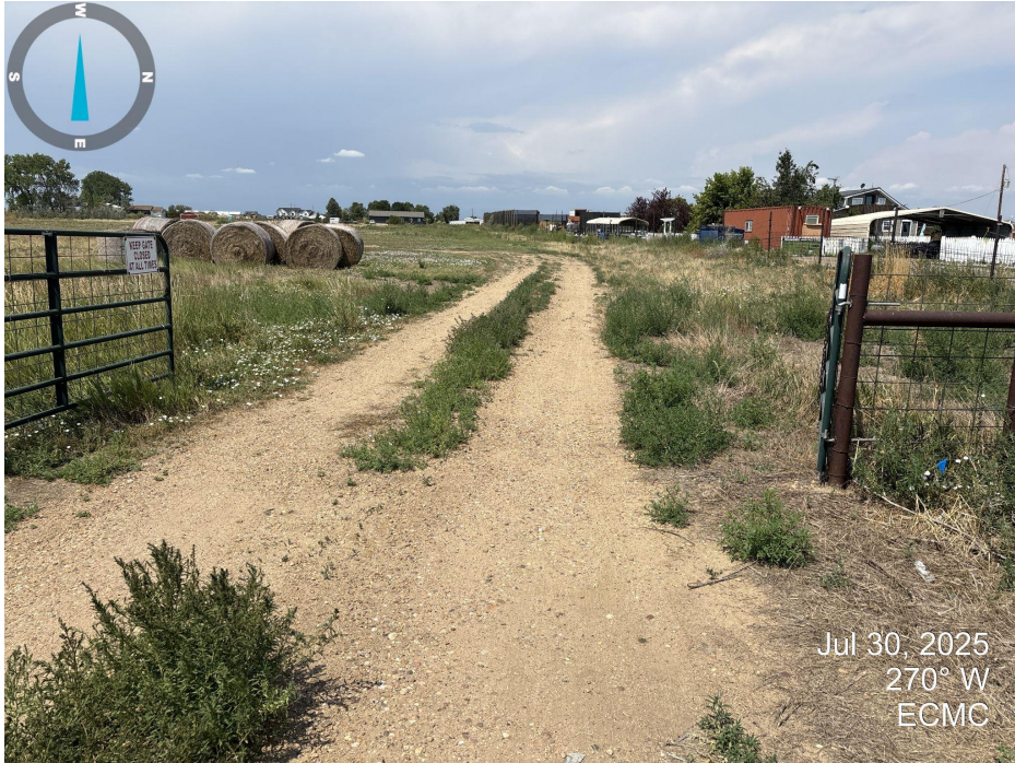
Photo 1. Looking west down the access road. It appears a new access road unrelated to oil and gas has been constructed partially overlapping the original access road.
