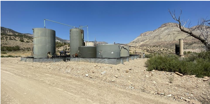
South West corner of location.
