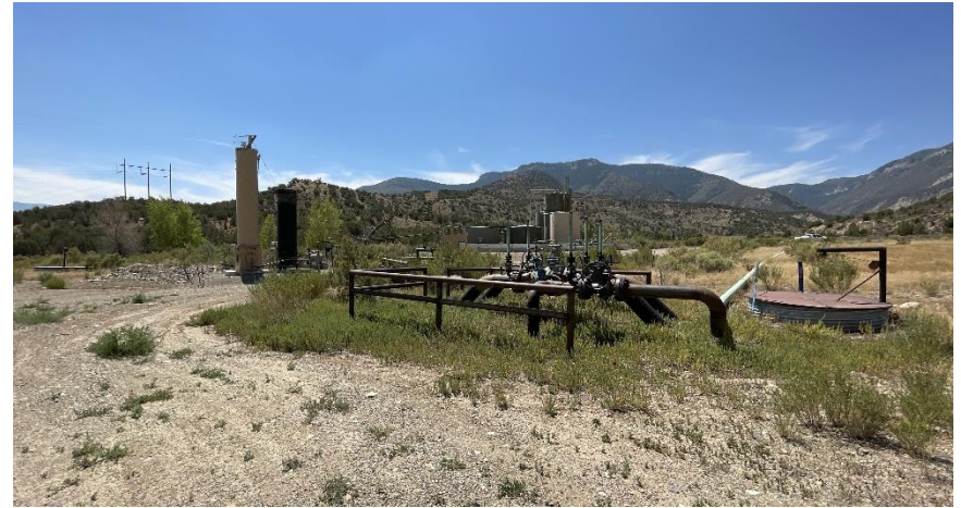
North East corner of location.
