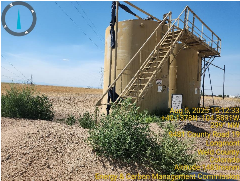
Photo 9 Tank Battery.
