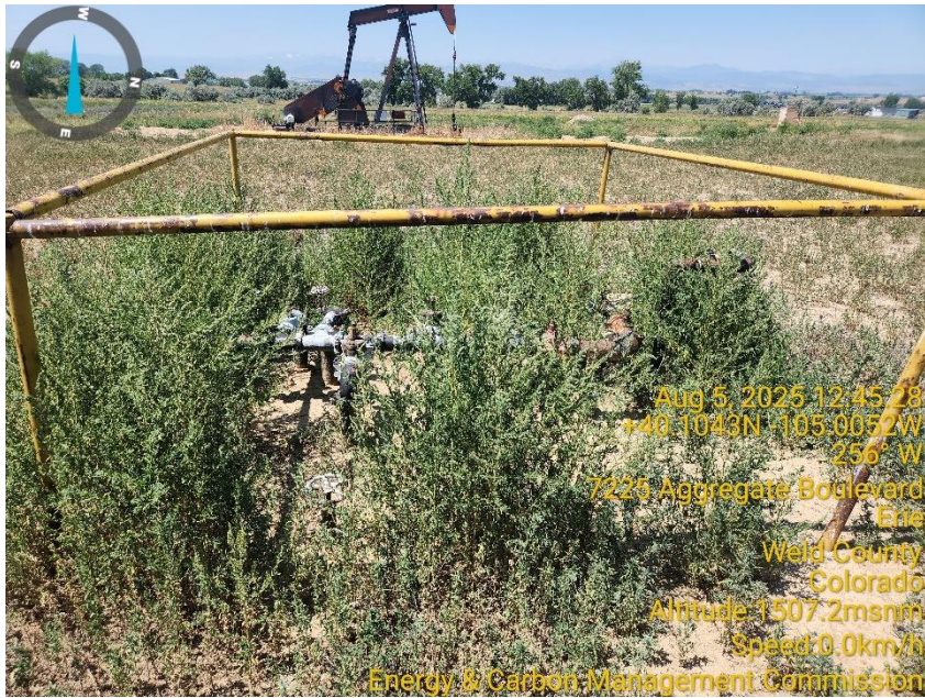
Photo 5 Flow line manifold in tall vegetation.
