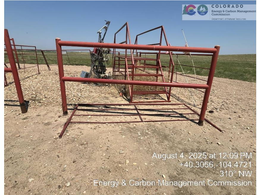
Unused Panel Fence
