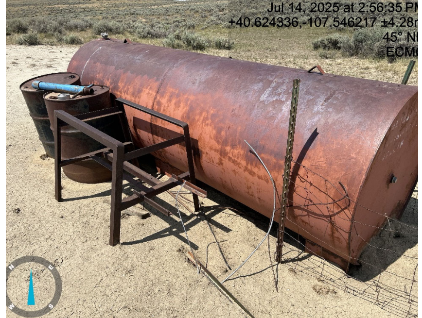
Unused equipment not contained/ debris
