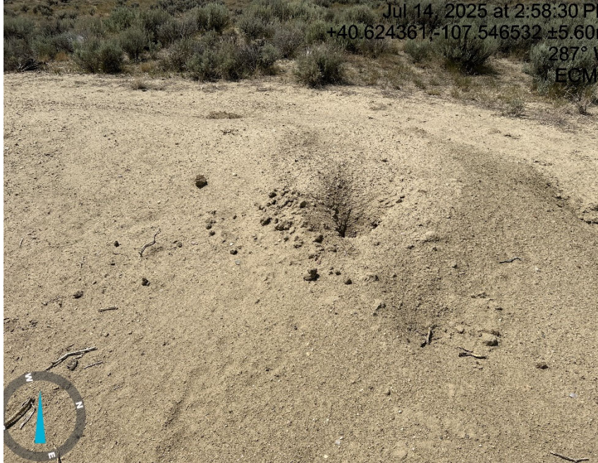
Holes in containment
