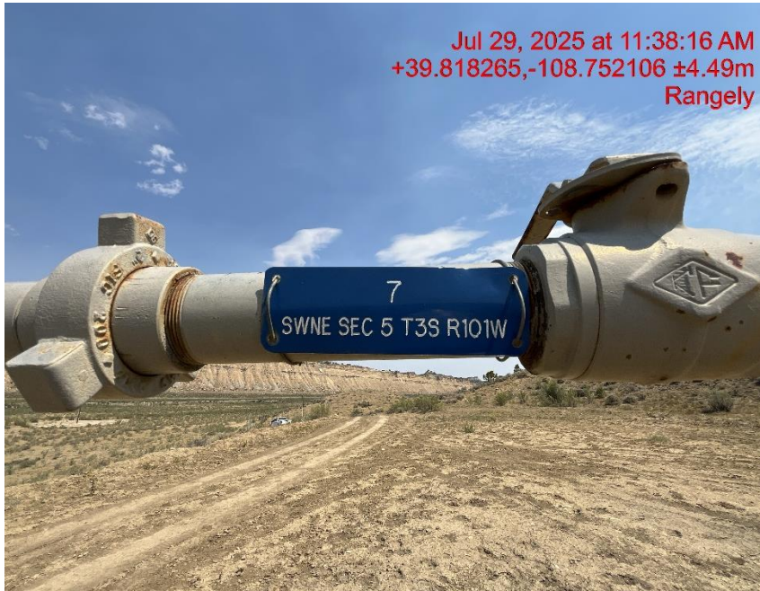
Photo # 0931 Wellhead sign lacks required information
