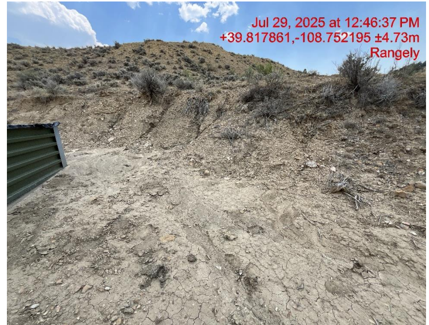
Photo # 0963 Failure to minimize erosion & transport of sediment - Erosion & transport of sediment on cutslope/sediment migrating onto location/insufficient BMP's
