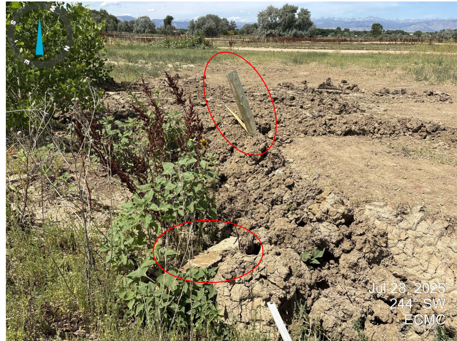
Photo 2. Looking west across the meter shed area. A depression/hole is present around the meter shed area.
