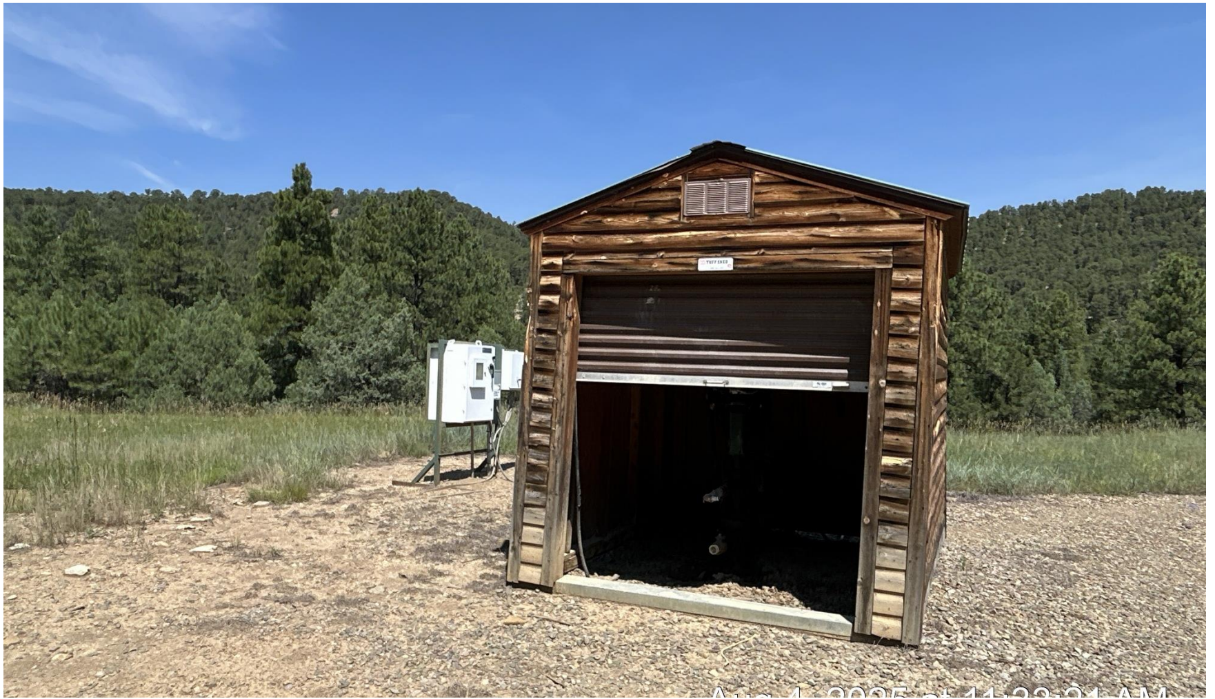
PHOTO 3: WELLHEAD AND EQUIPMENT
