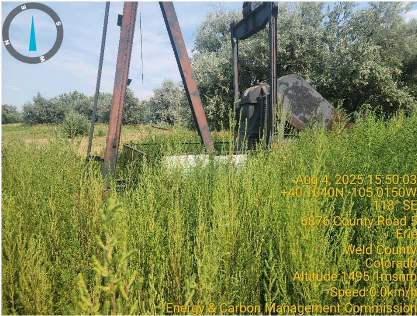
Photo 3 Wellsite sign over run with tall vegetation.
