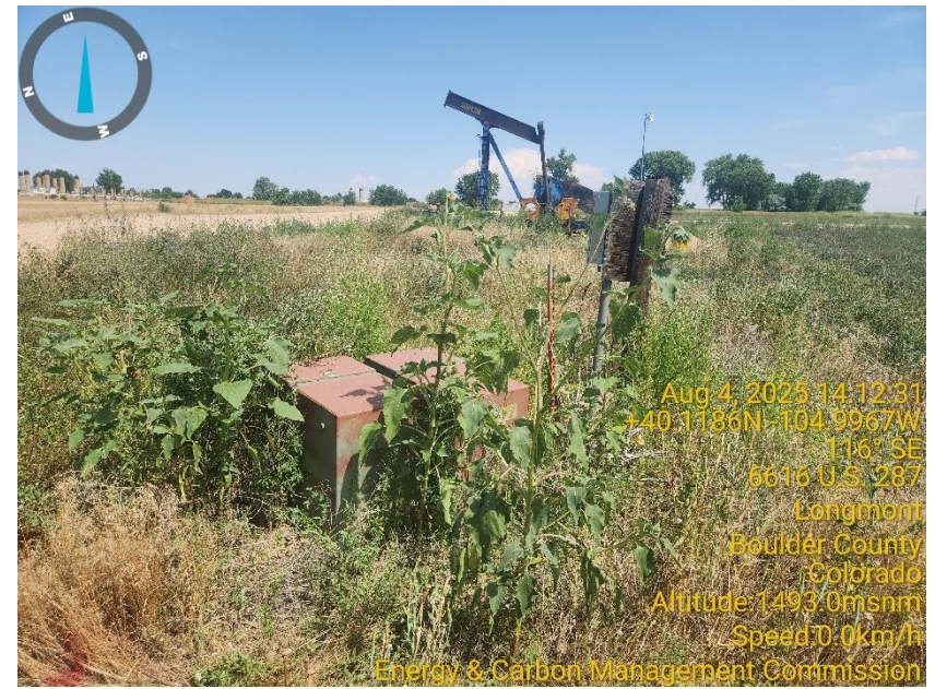
Photo 6 Meter box & transformers in the weeds.
