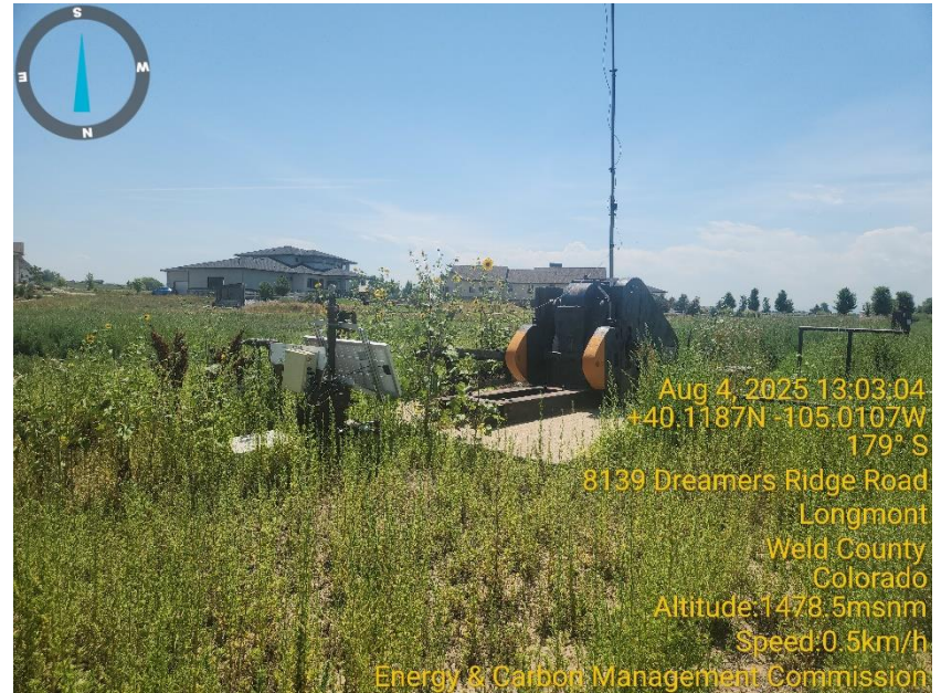
Photo 2 Unused pump jack.
