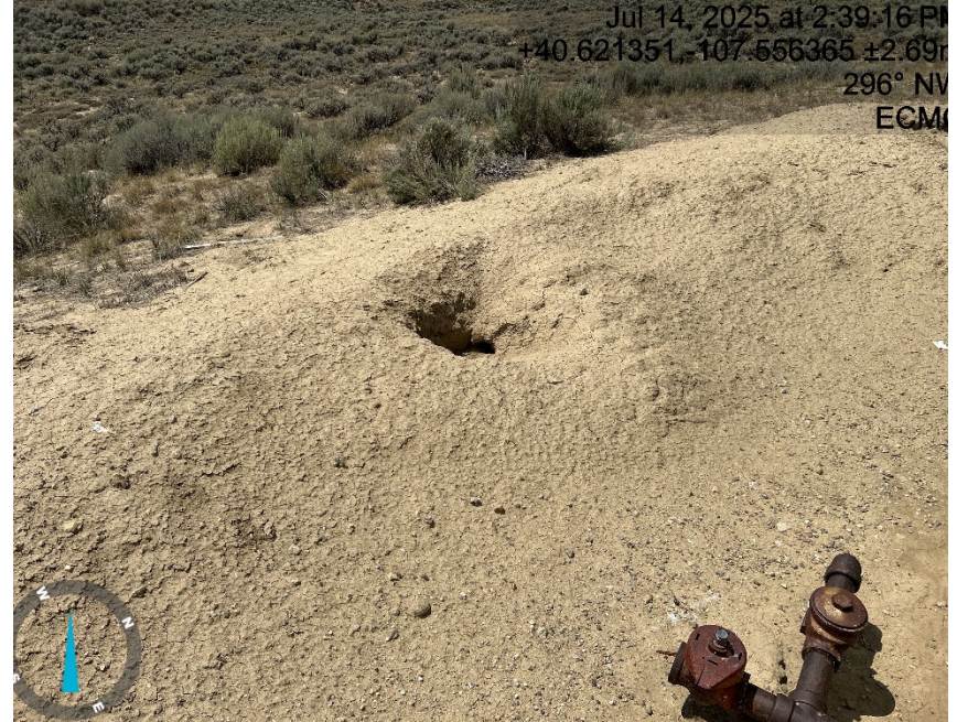
Holes in containment
