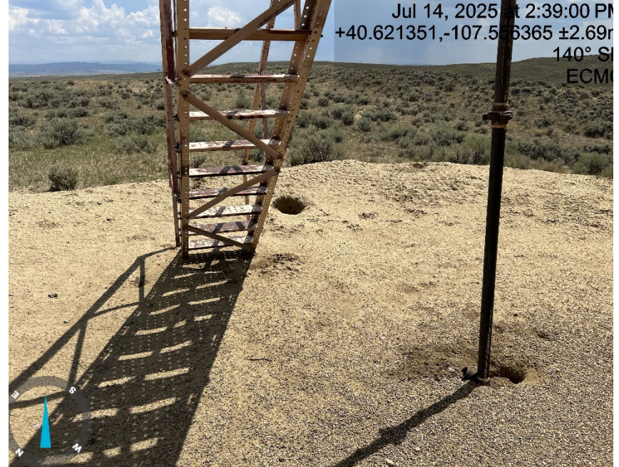
Holes in containment
