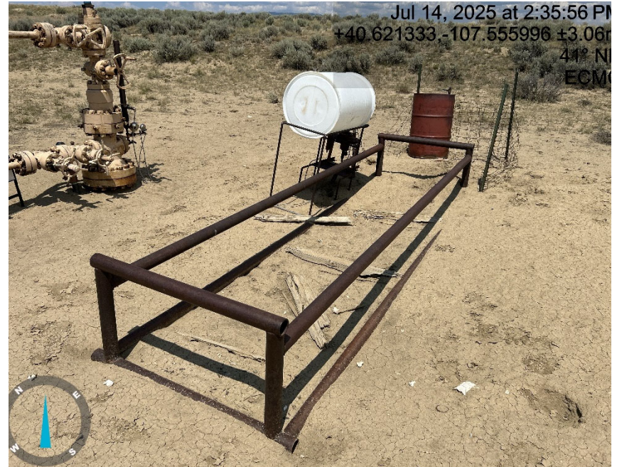
Debris and unused/ unmarked drums not contained
