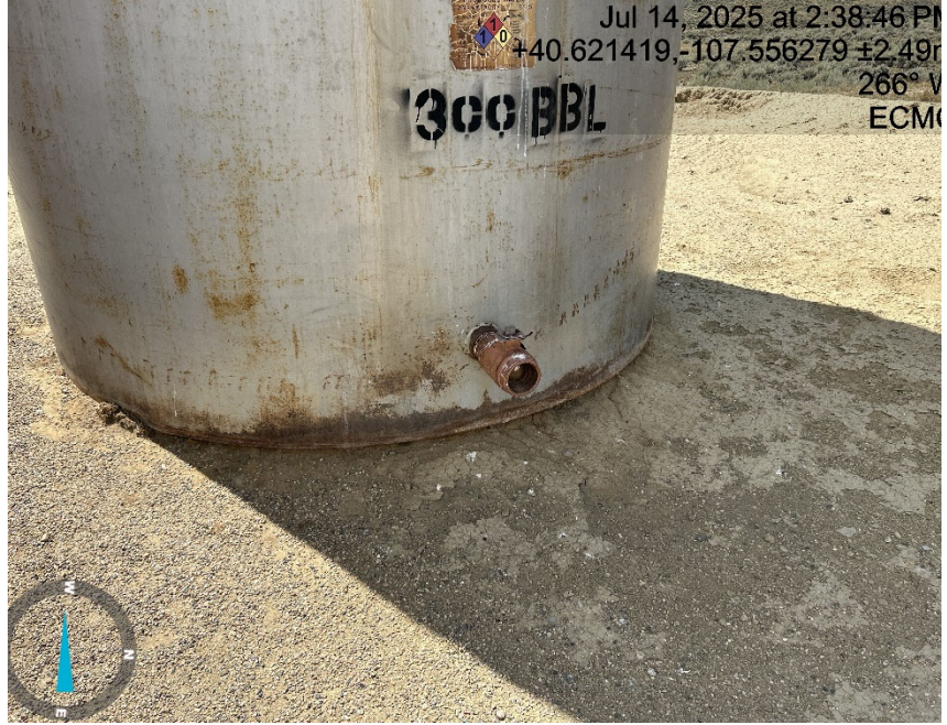
Open load line
