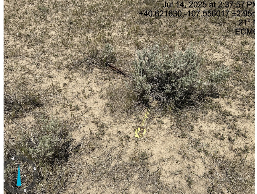
Dead man not marked properly
