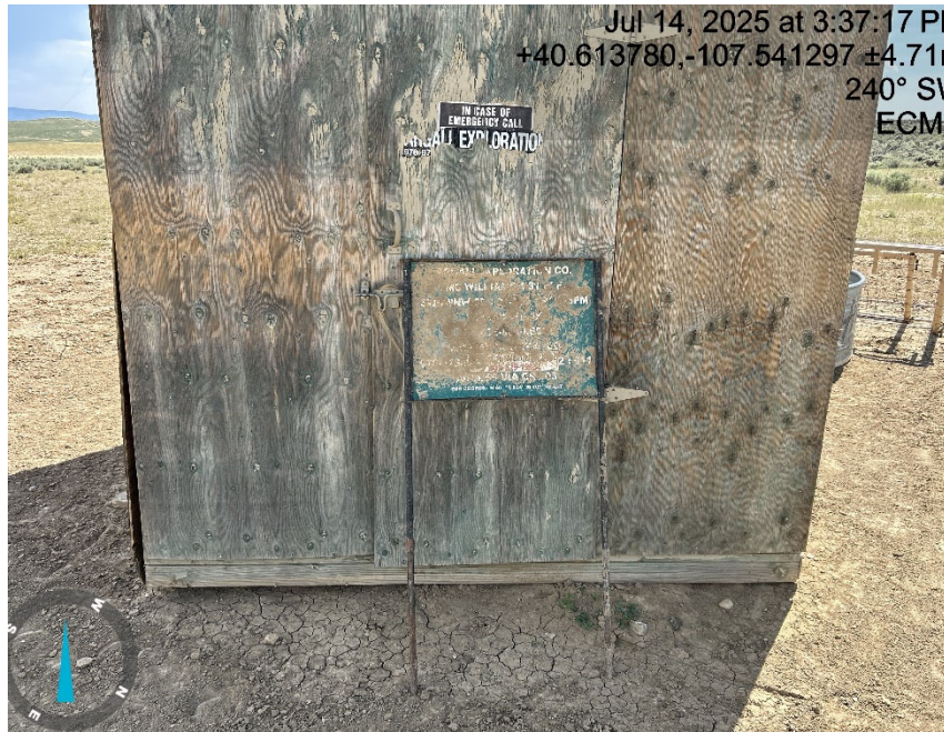
Well signage not legible.
