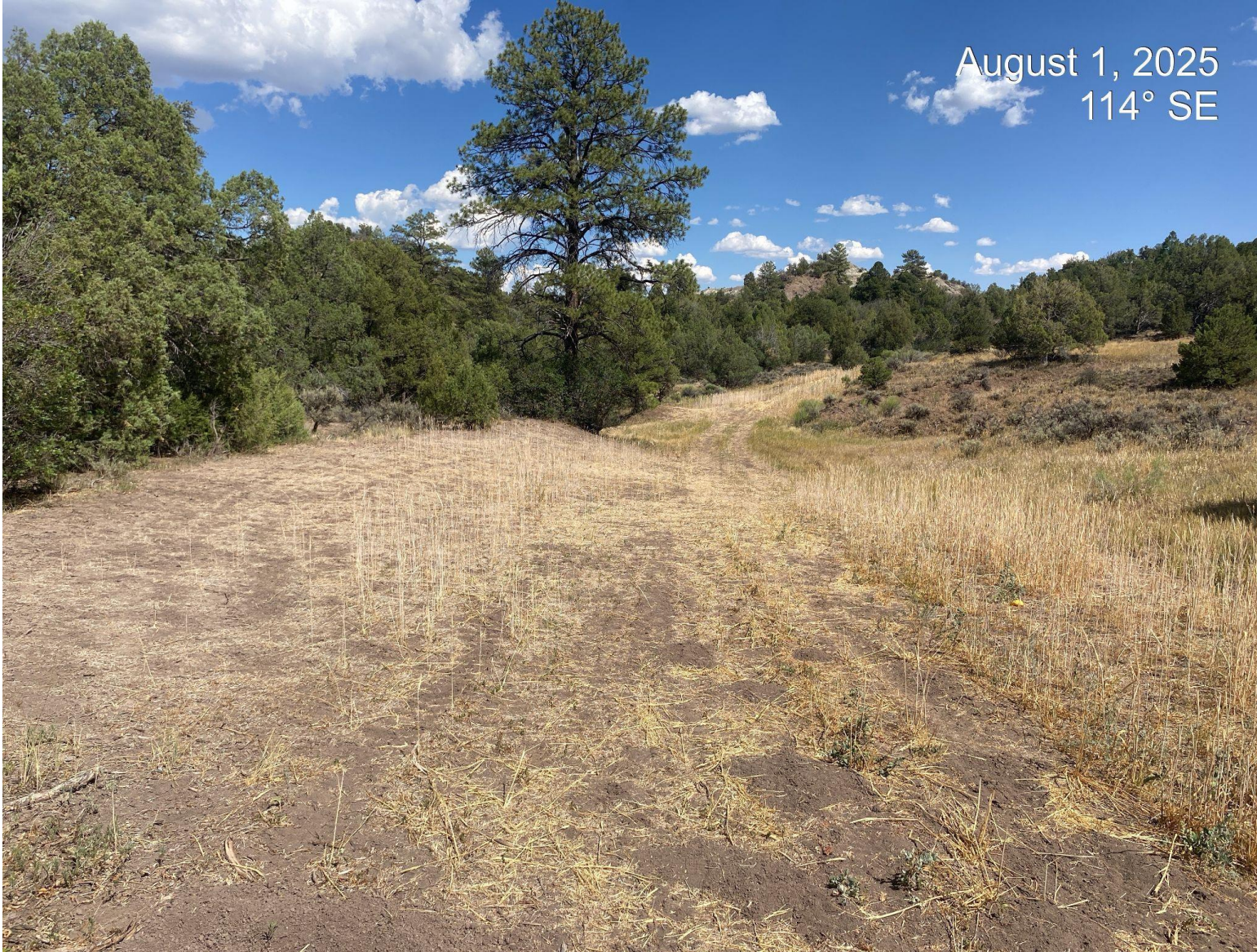
Photo 5. View of recently reclaimed access road taken from the starting point facing south towards reclaimed well pad.
