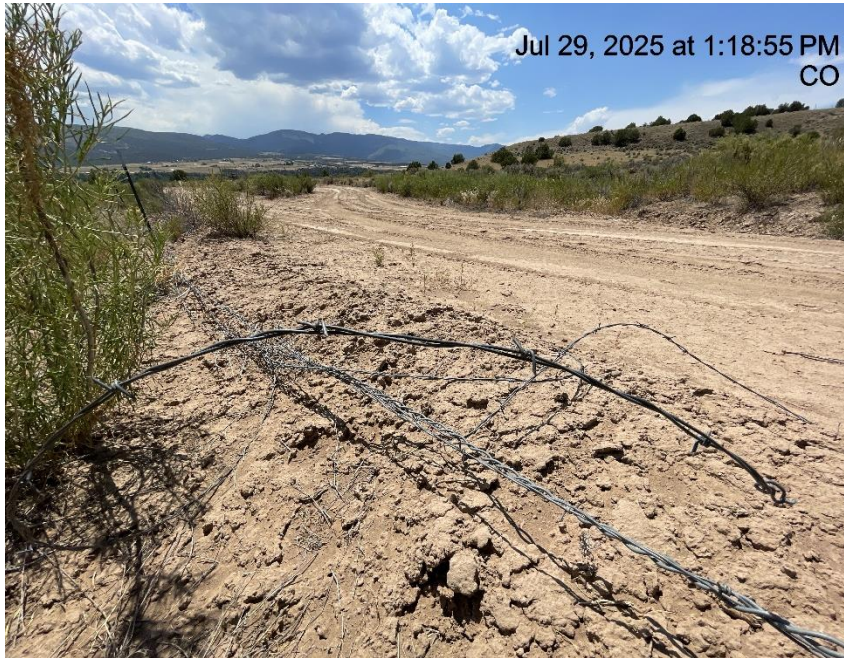
Photo # 5697 Barbed wire fence needs maintenance/wildlife hazard
