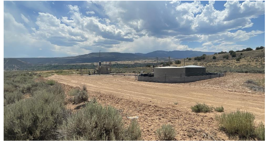
North East corner of location.
