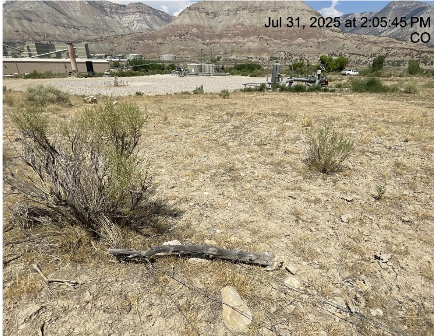
Photo # 6397 Barbed wire fence needs maintenance/wildlife hazard
