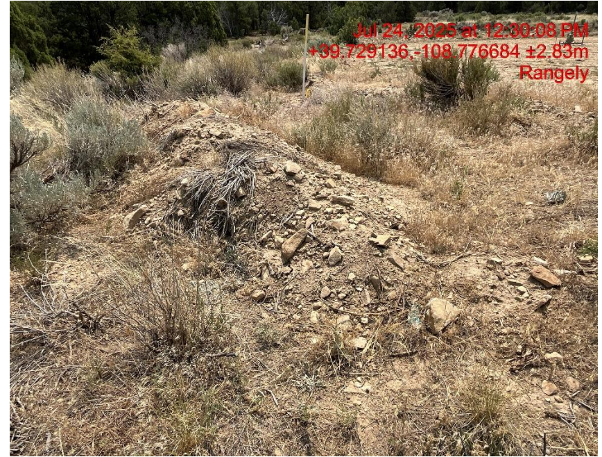
Photo # 0868 Stockpiled soils with no BMP's
