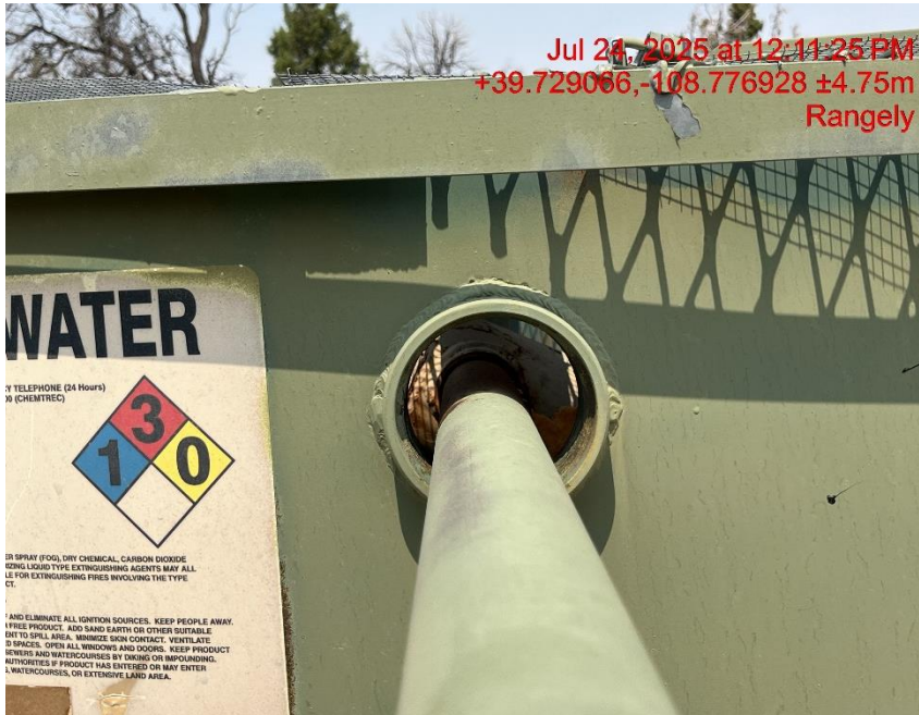
Photo # 0853 Open port on production tank/wildlife hazard/available for entry by wildlife
