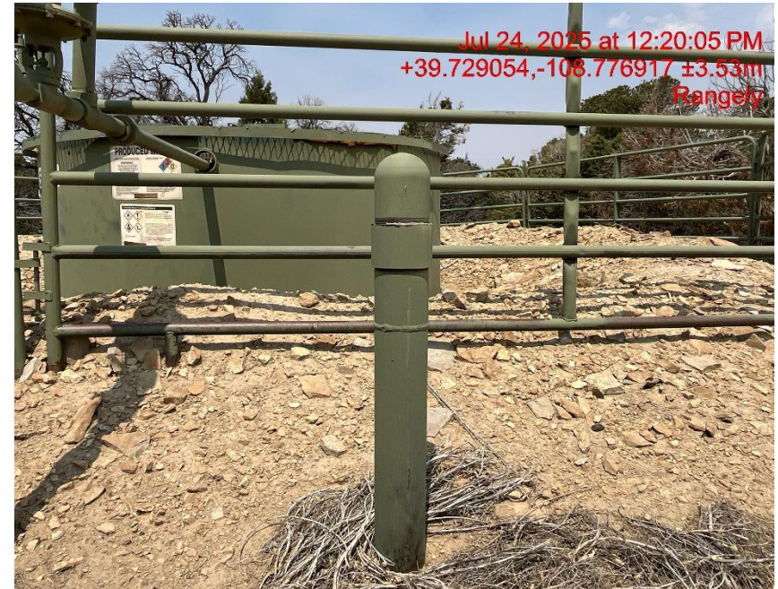
Photo # 0858 Unused flowline does not comply with CECMC 600 & 1100 series rules
