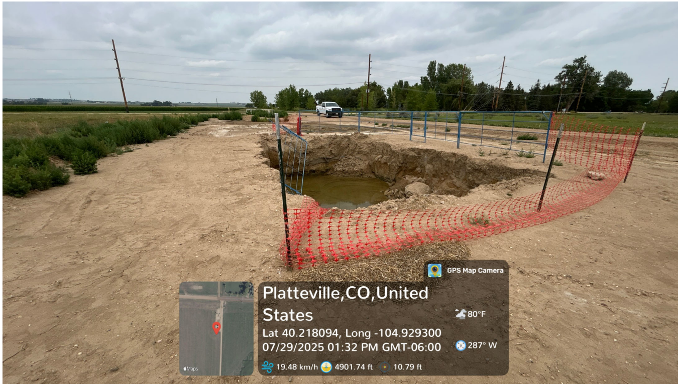
Photo 5 – Facing Northeast towards open excavation
