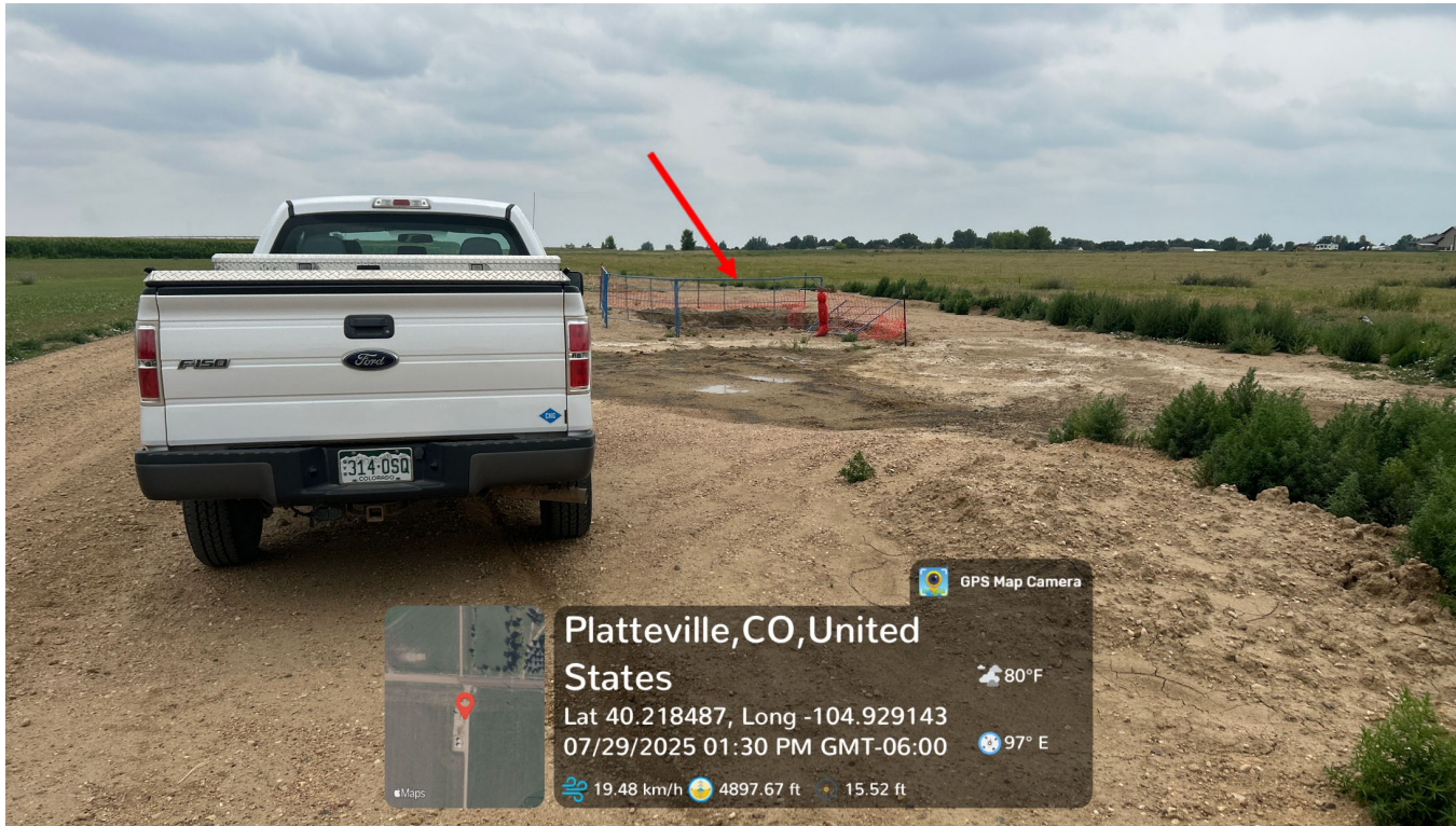
Photo 1 – Facing Excavation from County Road 32 facing South
