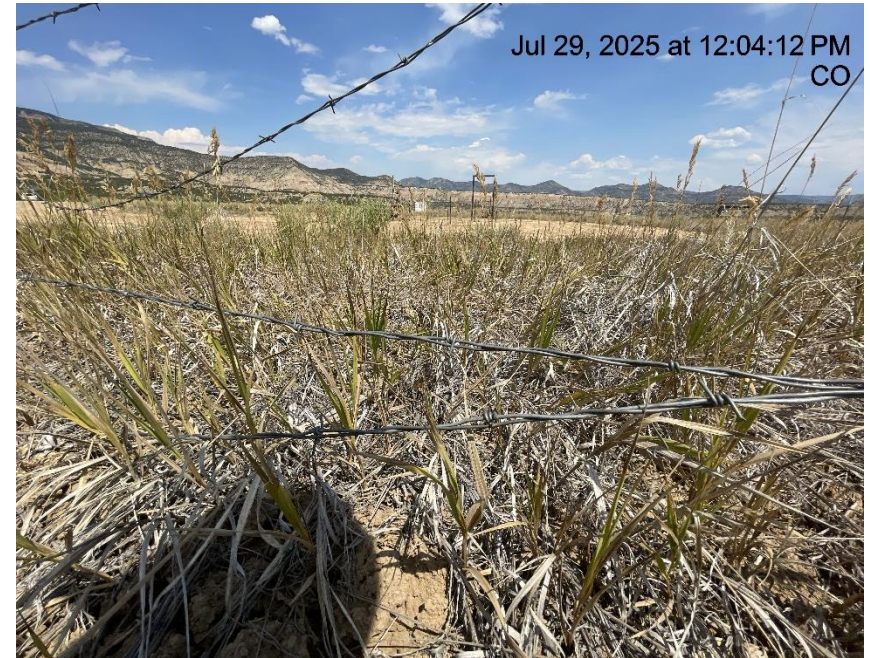
Photo # 5490 Barbed wire fence needs maintenance/wildlife hazard
