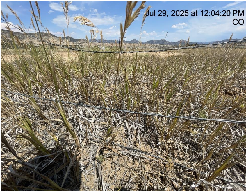
Photo # 5491 Barbed wire fence needs maintenance/wildlife hazard
