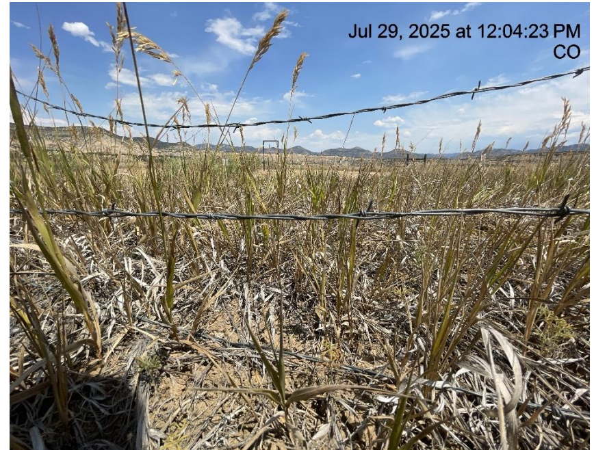
Photo # 5492 Barbed wire fence needs maintenance/wildlife hazard
