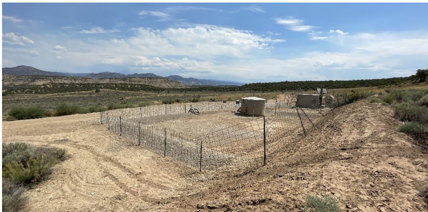
South West corner of location.
