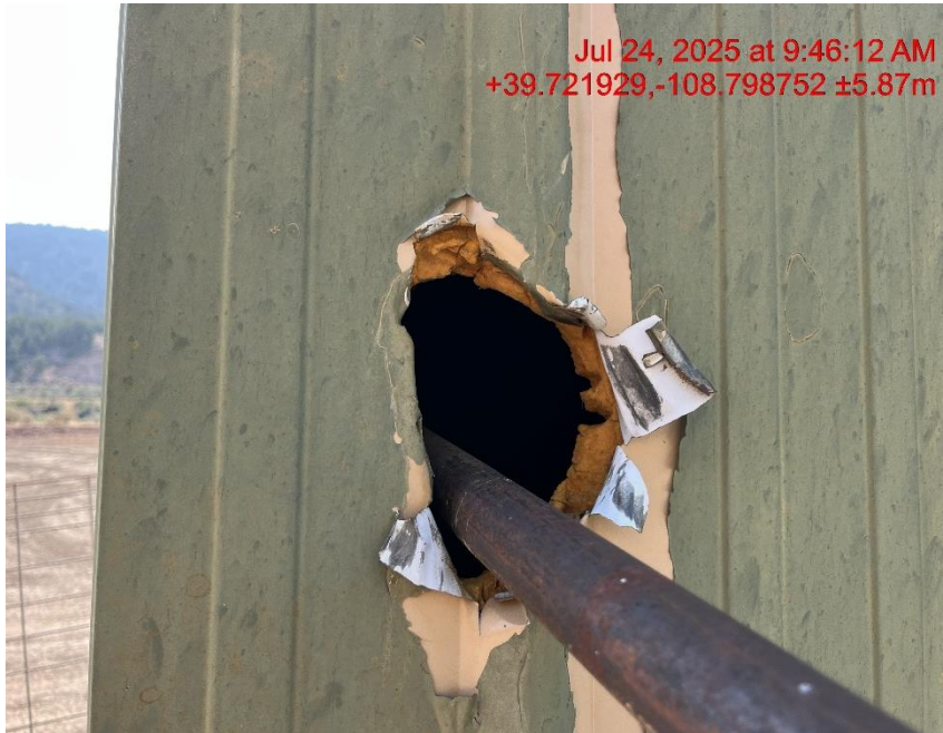
Photo # 0784 Hole in meter house open to wildlife/available for entry by wildlife
