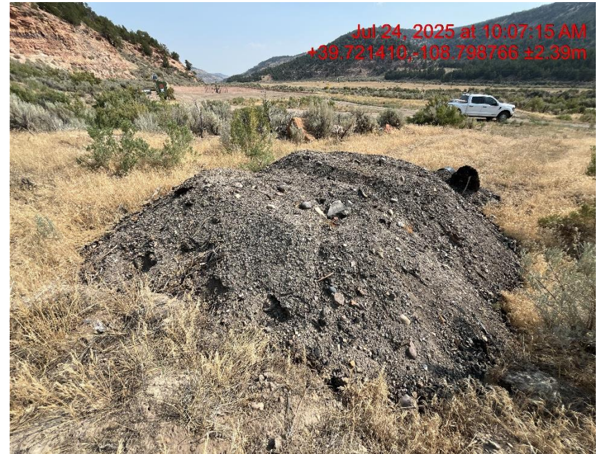
Photo # 0798 Stockpiled soils with no BMP's
