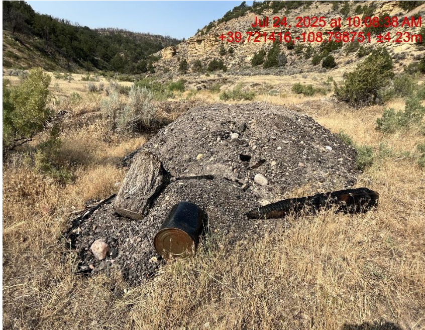
Photo # 0800 Stockpiled soils with no BMP's
