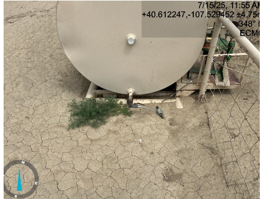
Stored equipment/ Debris
