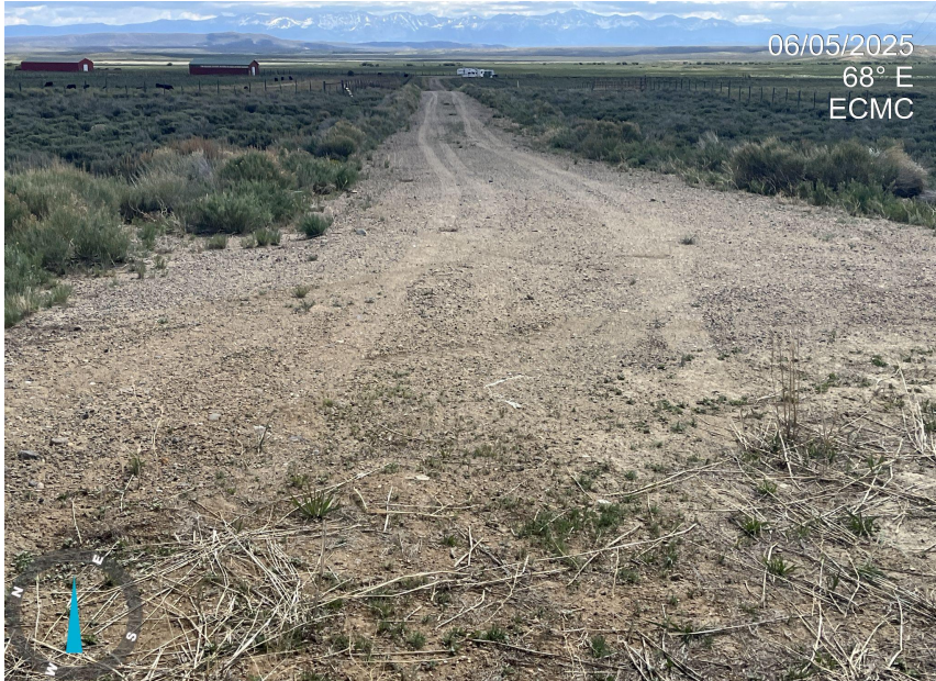
Photo 5. Photo taken of the access road from the entrance of the Location, facing east. The access road has not been recontoured, removed of gravel, alleviated of compaction or re-seeded. Reclaim the access road per 1004.a. and 1004.d.
