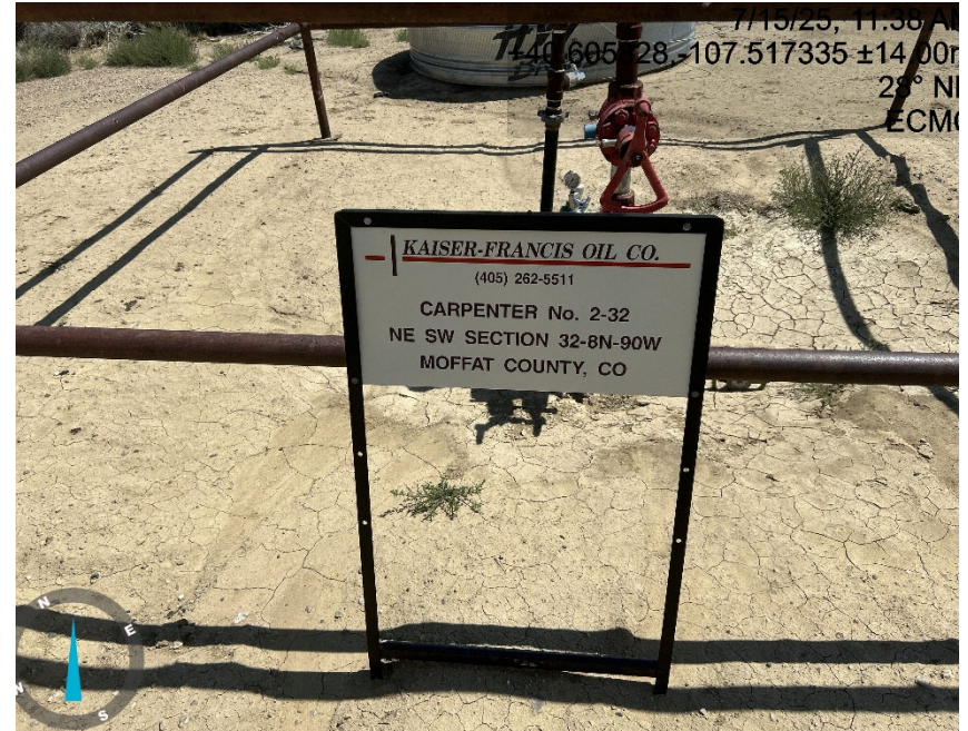
Well signage lacks information
