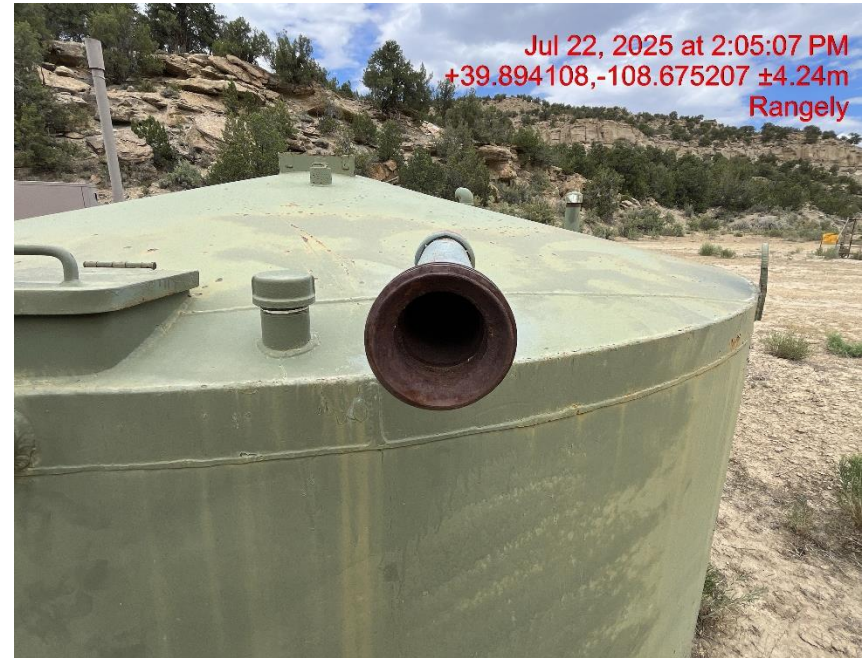
Photo # 0613 Open ended piping on tank/wildlife hazard/available for entry by wildlife
