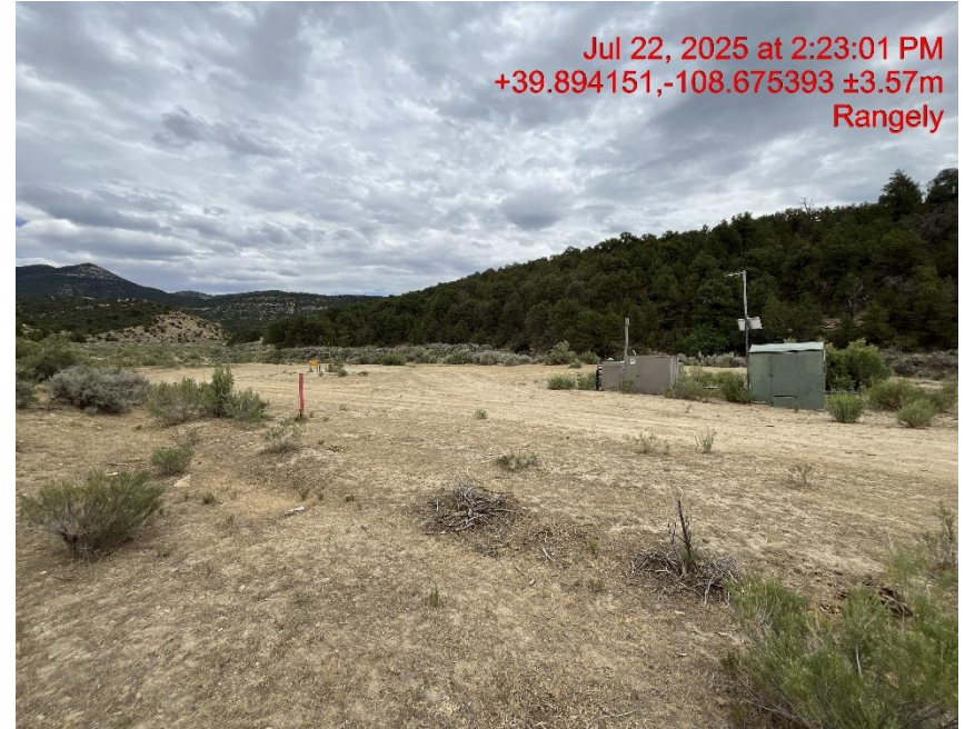
Photo # 0631 NW corner of location
