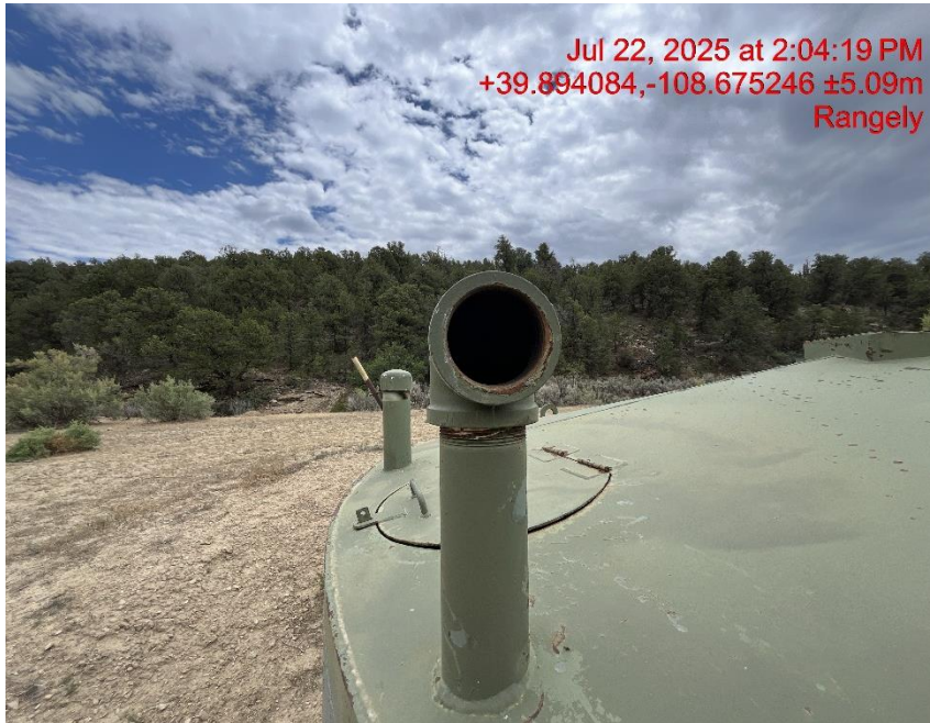
Photo # 0612 Open ended piping on tank/wildlife hazard/available for entry by wildlife
