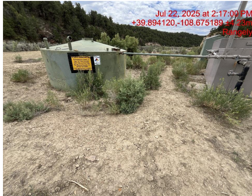
Photo # 0622 Weeds/undesirable plant species surrounding production equipment constitutes a fire hazard
