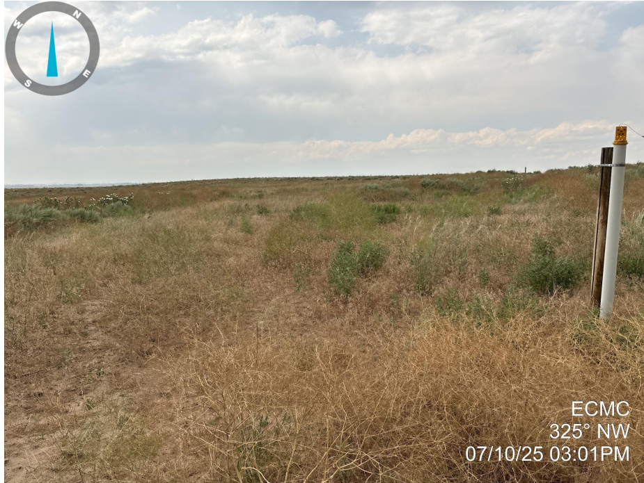
Photo 7. Photo taken of the access road to the location, facing northwest. Photo illustrates midstream equipment remains along the access road.
