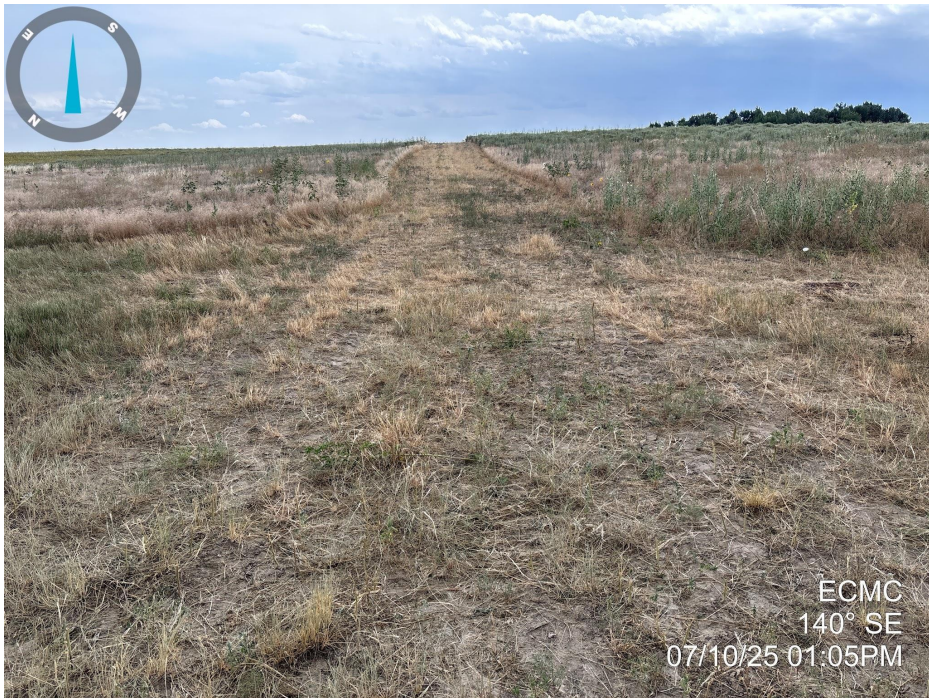
Photo 5. Photo taken of the access road to the location, facing southeast, away from the location. Photo illustrates that final reclamation activities have taken place, but vegetation establishment does not meet Rule 1004 standards. The site has been recently mowed and cheatgrass ( Bromus tectorum ), a List C Noxious Weed species, was observed across the access road.
