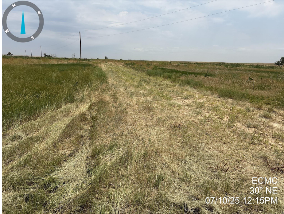
Photo 7. Photo taken of the access road to the location, facing northeast. See comments under Photo 6.
