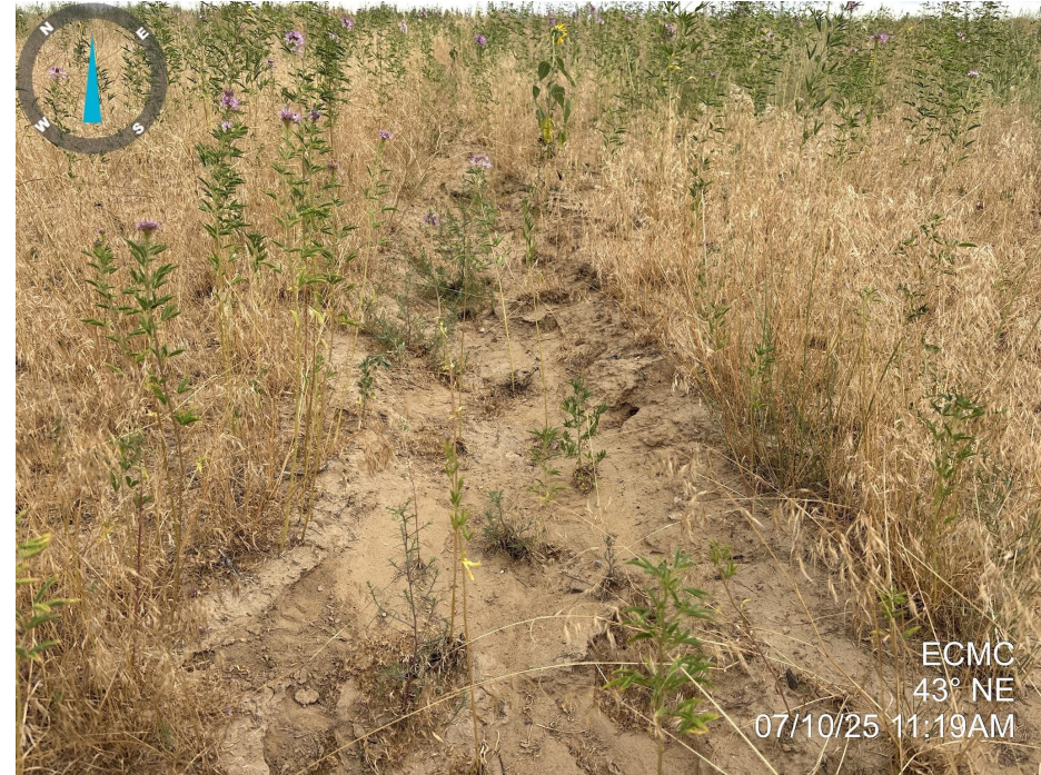
Photo 6. Photo taken of the access road to the well location, facing northeast. Photo illustrates stormwater erosion along portions of the access road.
