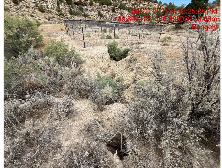
Photo # 0562 Failure to minimize erosion & transport of sediment off location/insufficient BMP's
