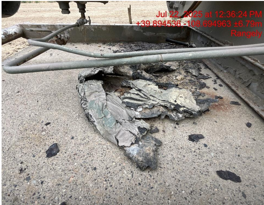
Photo # 0568 Debris on location
