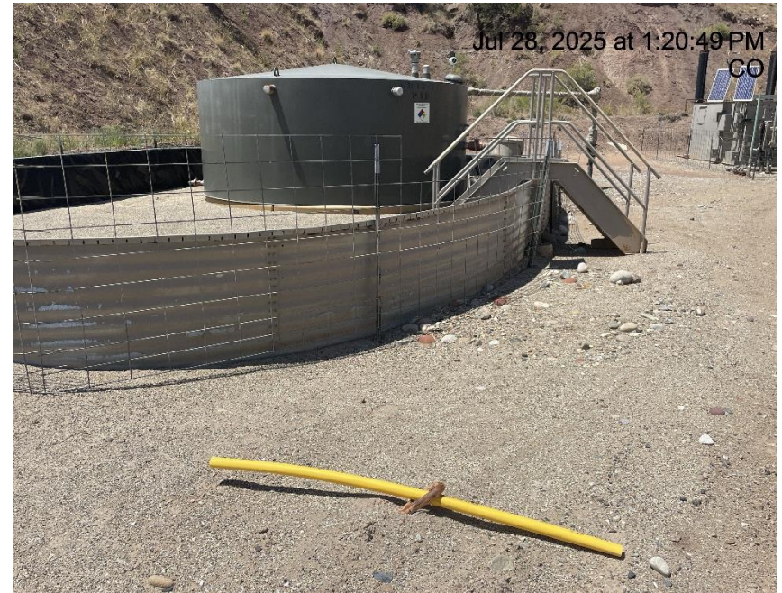
Photo # 5242 Same improperly marked deadman
