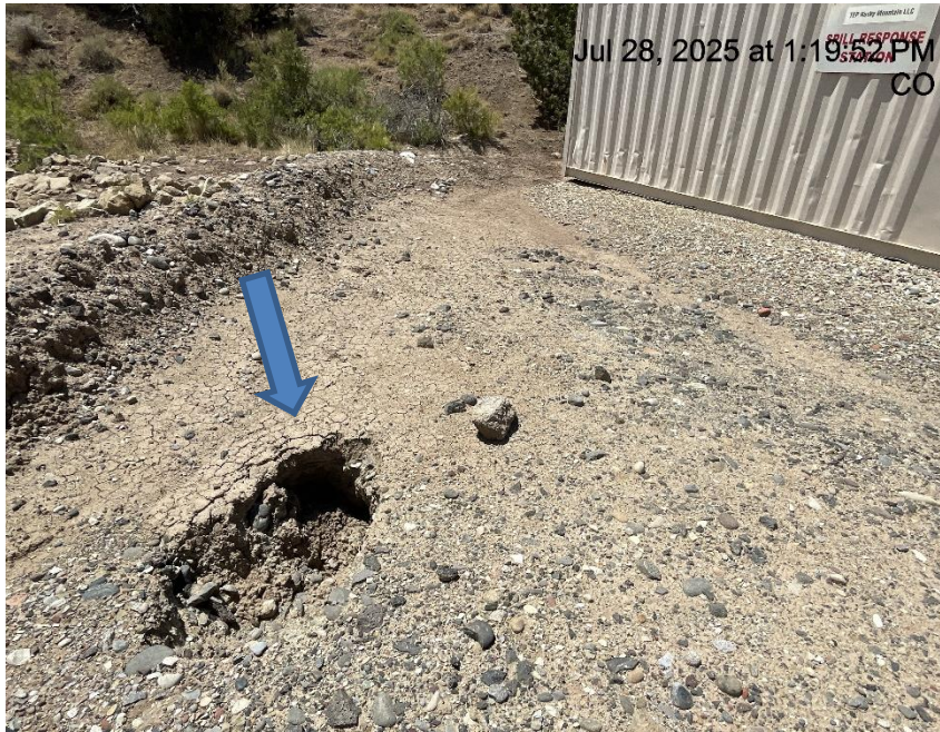
Photo # 5245 Subsidence on location (additionally this is also a wildlife & personnel hazard)
