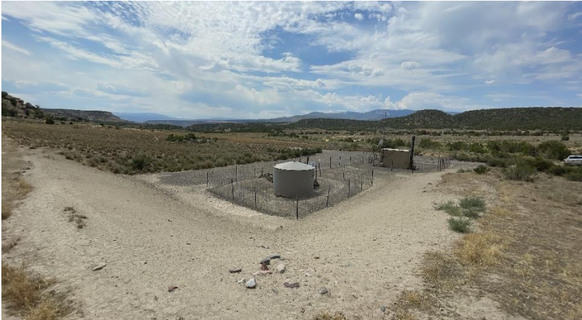
North West corner of location.
